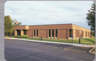
Headquarters Willowbrook, Illinois.
